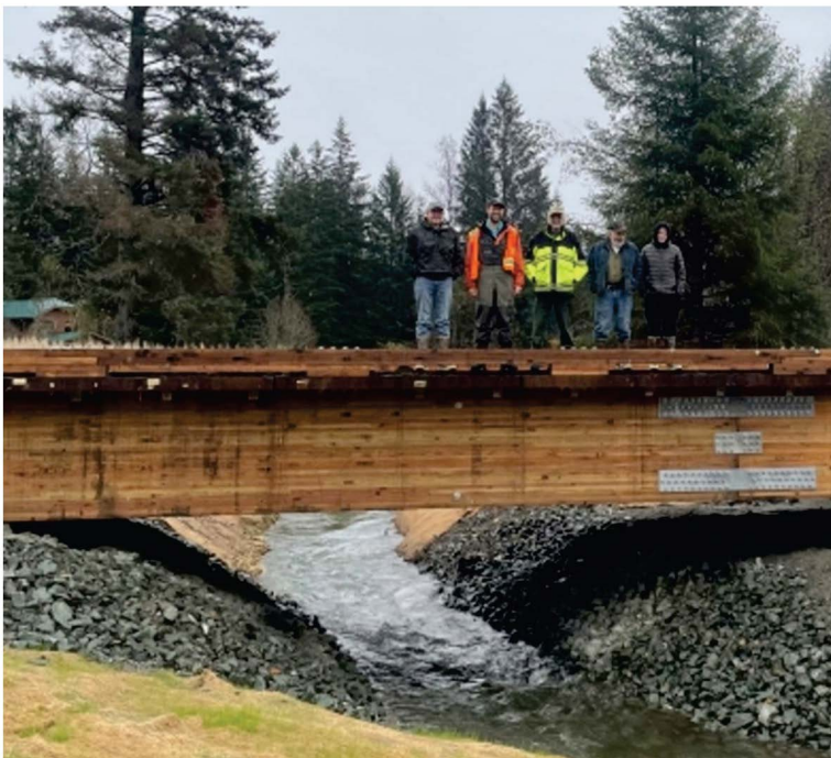
The new bridge as of October 2022.
