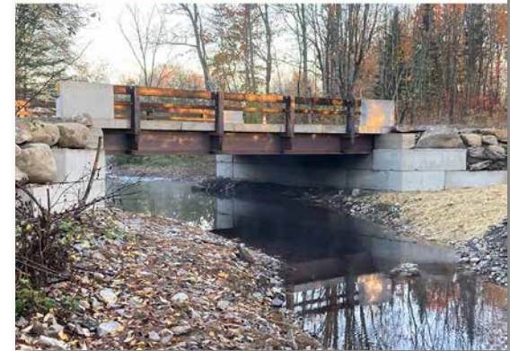
Perched culverts (top) are impassible by fish and other aquatic life. This newly constructed bridge (bottom) in the Town of Charleston, ME will allow aquatic life to reconnect with upstream habitats. Photo credit: USFWS
