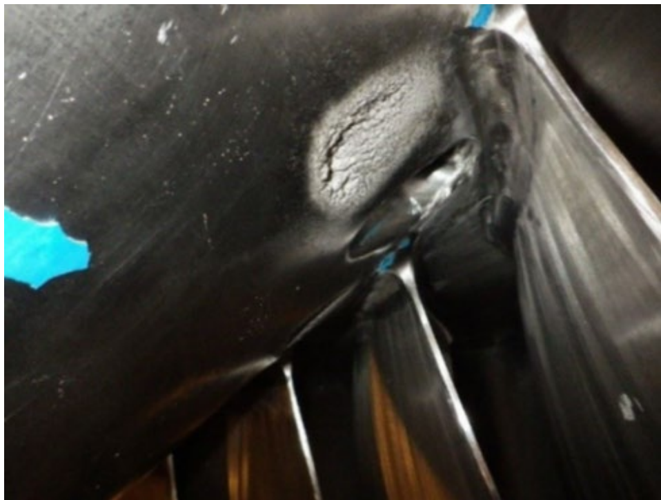
TURBINE RUNNER DAMAGE FROM CAVITATION (SOURCE: BUREAU OF RECLAMATION)
