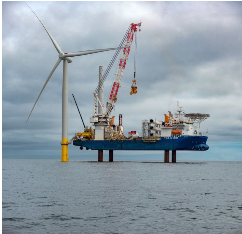
CRANE INSTALLING AN OFFSHORE WIND TURBINE (SOURCE: BSEE RENEWABLE ENERGY PROGRAM)
