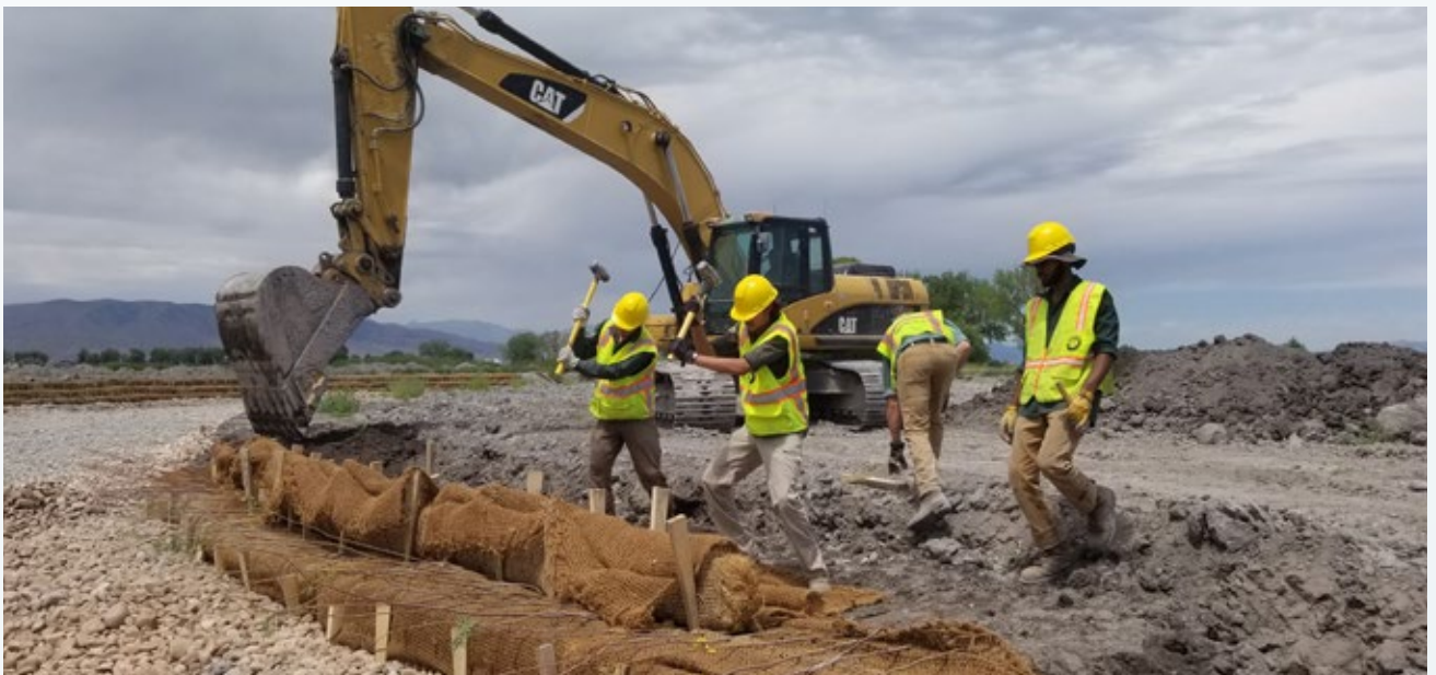
Stream bank construction on the Provo River Delta.
