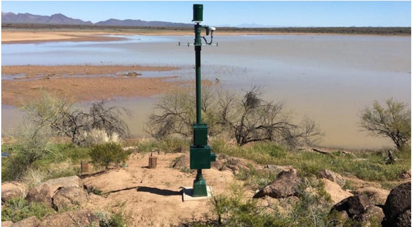
Early warning systems site at Menagers Dam, Tohono O'odham Nation.
