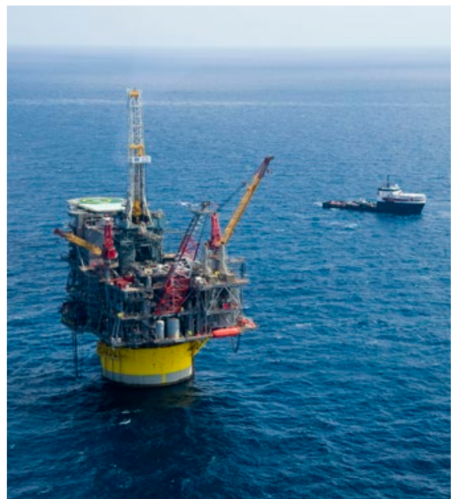
A deepwater offshore production platform, Gulf of Mexico.
