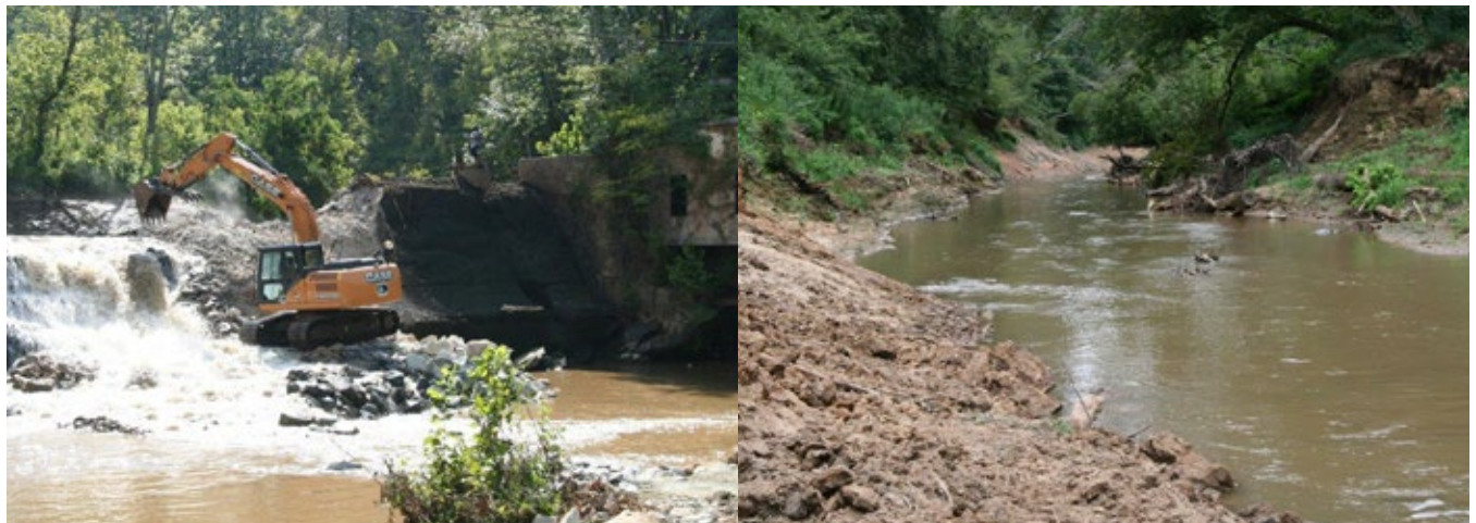
As part of the restoration activities for the Dan River Coal Ash Spill NRDAR case, the Pigg River Dam in Virginia was removed to return riverine conditions to 2.2 miles of the formerly impounded reach and restore fish passage for game fish such as smallmouth bass and other nongame fish, such as the federally and state listed endangered Roanoke logperch.
