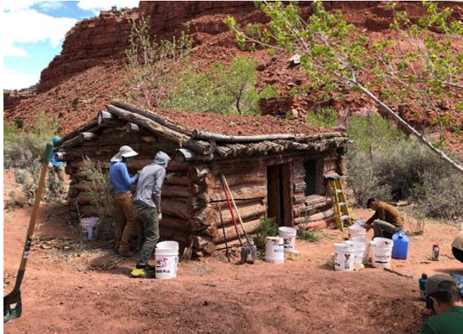
Volunteers work on restoring the roofing and chinking of Watson Cabin.
