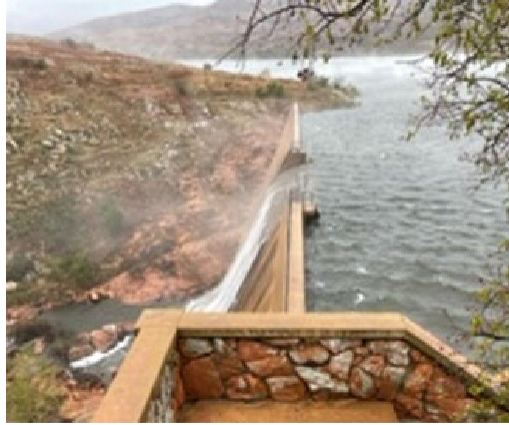
Significant rain event at Lake Jed Johnson Dam, Wichita Mountain Wildlife Refuge, Oklahoma, October 2023.
