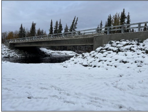
After photo of brand new concrete girder bridge at Sourdough Campground. Photo Credit: Curt Fortenberry
