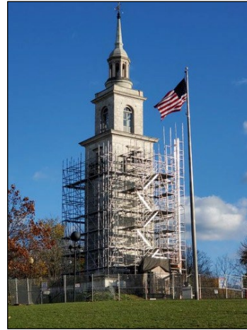
Stabilization work on Dorchester Heights Monument. Photo Credit: NPS
