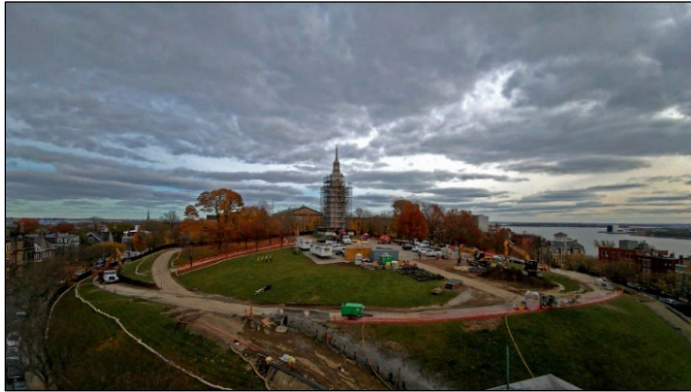
Construction at Dorchester Heights Monument. Photo Credit: NPS
