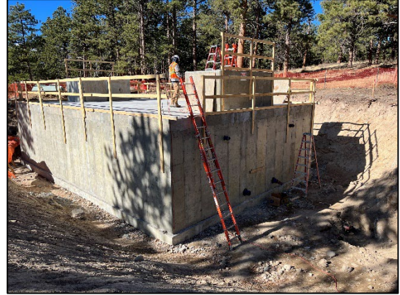
Construction of a water tank. Photo Credit: NPS DSC project team
