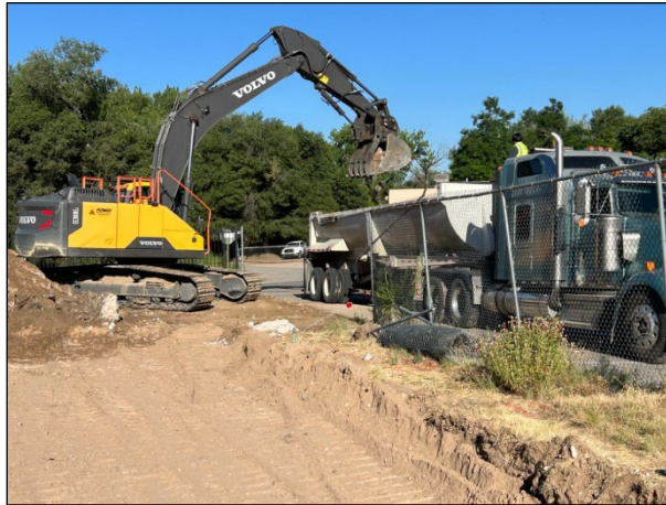
Construction work at Ohkay Owingeh Community School. Photo Credit: BIE
