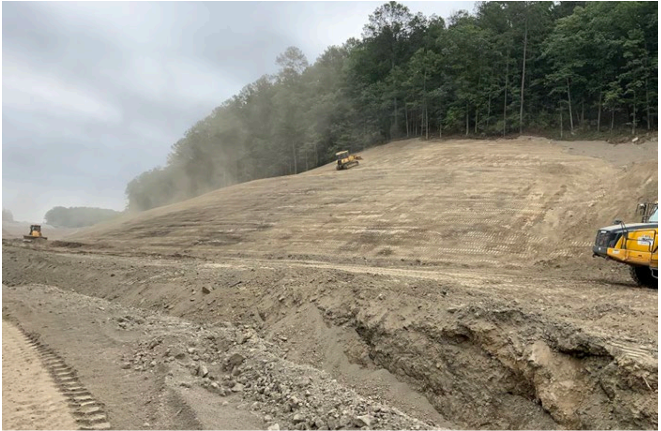
Piper Mine Reclamation Project on the Cahaba National Wildlife Refuge, AL.
