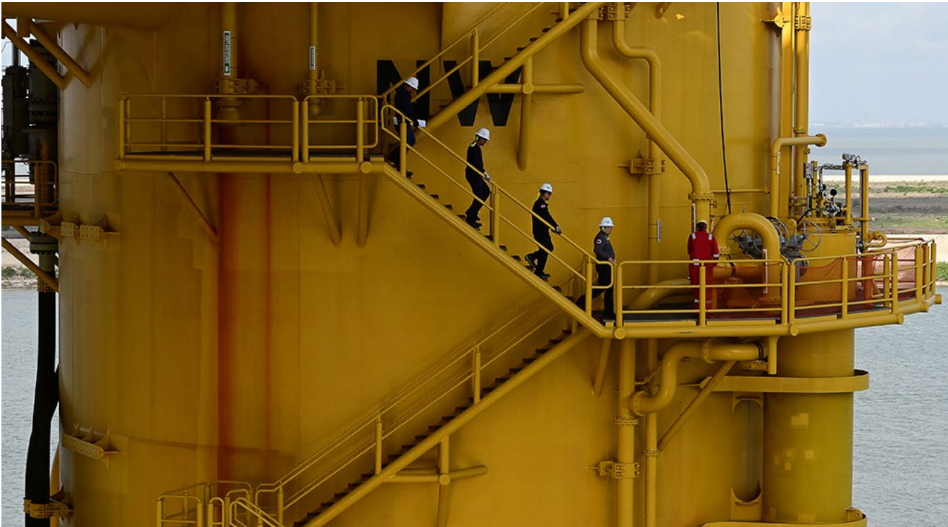
BSEE conducts pre-production inspection on a platform in Texas.
