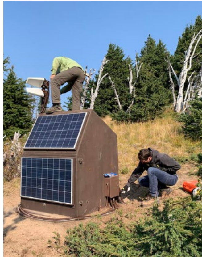
A USGS Cascades Volcano Observatory field team finishes the installation of the combined seismic/GPS station at Mount Hood, OR.
