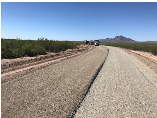
Haekel Road under repair. Photo credit: BLM
