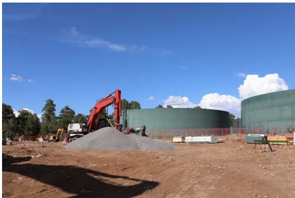
Construction at the South Rim Wastewater Plant. Photo Credit: NPS
