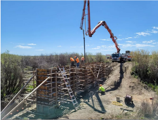
Construction in Camas NWR. Photo Credit: Cole Woodman, Global Engineering Services
