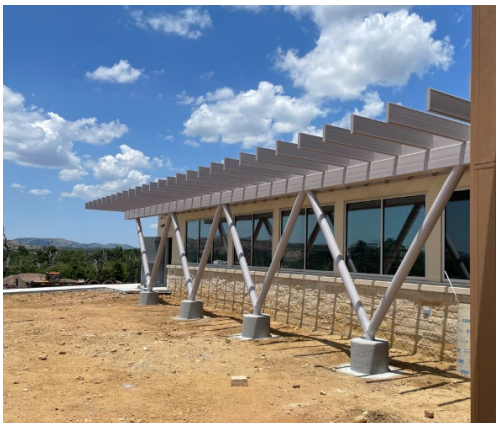
Repairs at Wichita Mountains Wildlife Refuge. Photo credit: FWS
