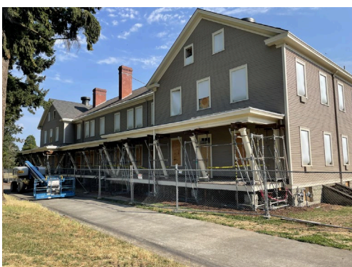
Repairs to Barracks Building. Photo credit: NPS
