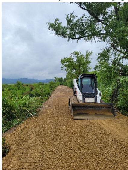
Trail at Trempealeau National Wildlife Refuge under construction. Photo Credit: USFWS
