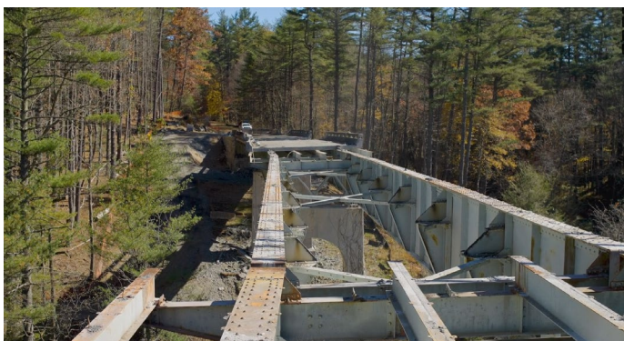
Blue Ridge Parkway's Laurel Fork Bridge under construction. Photo Credit: NPS
