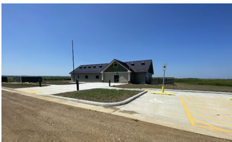
Completed headquarters at Lake Andes National Wildlife Refuge. Photo Credit: USFWS
