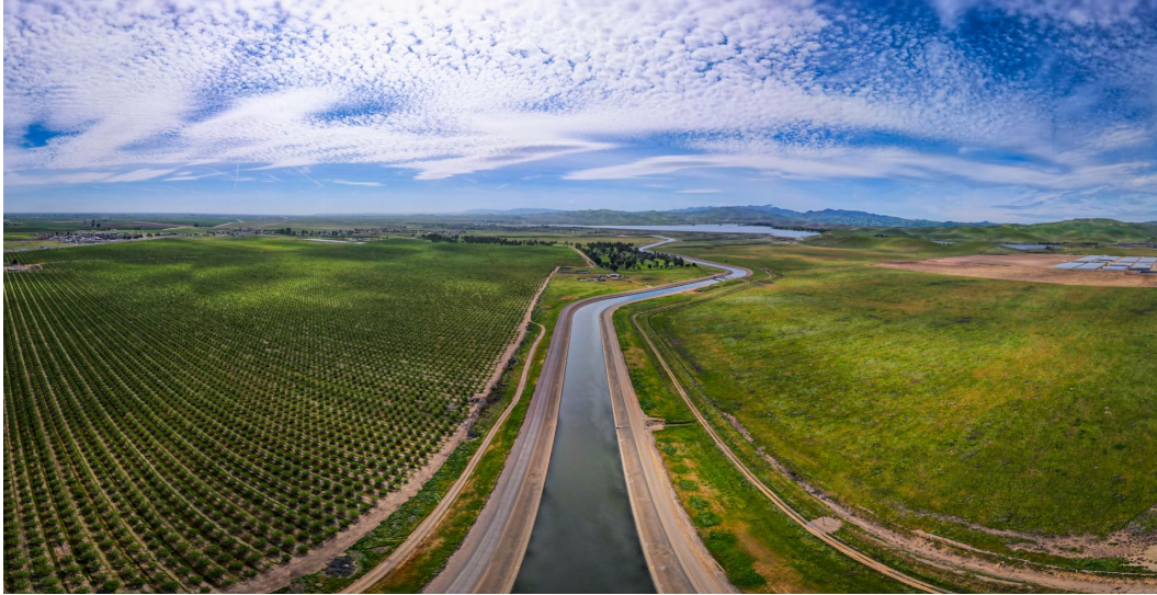
Figure 6 Innovative Solar Panel Installation over irrigation canals will decrease evaporation while advancing clean energy goals.
