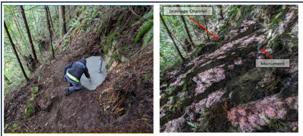
Left: Subsidence feature reclaimed using a PUF plug with a steel mesh-reinforced concrete veneer. Photo taken on November 8, 2023. Right: Completed site restoration at the subsidence feature. Photo taken November 13, 2023. Photos taken by OSMRE Project Manager Cody Yankey.
