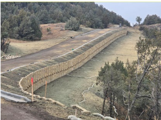
Completed log pile retaining wall, prior to repaving at Theodore Roosevelt National Park. Photo Credit: NPS
