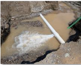
Broken pipe in the Furnace Creek water system, Death Valley National Park. Photo Credit: NPS
