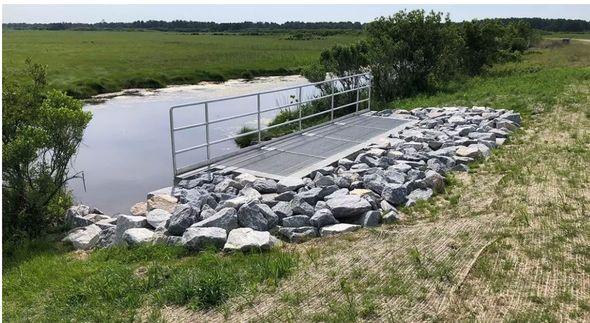
Wetland managers use water control structures like this one to help regulate water levels to control exotic invasive vegetation at Cedar Point and Ottawa National Wildlife Refuges in Ohio. Photo: USFWS.
