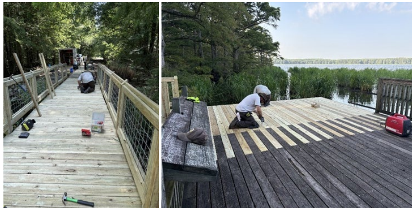
GAOA Funded Maintenance Professionals Repairing a Damaged Fishing Pier at Wappanocca NWR. Image: USFWS
