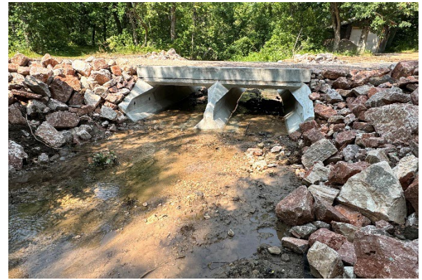
Photo Caption: Newly replaced creek crossing at the Alkali Creek Campground
