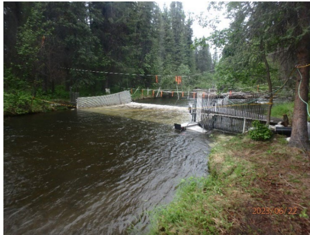
Tanada Creek Salmon Weir, 2023
