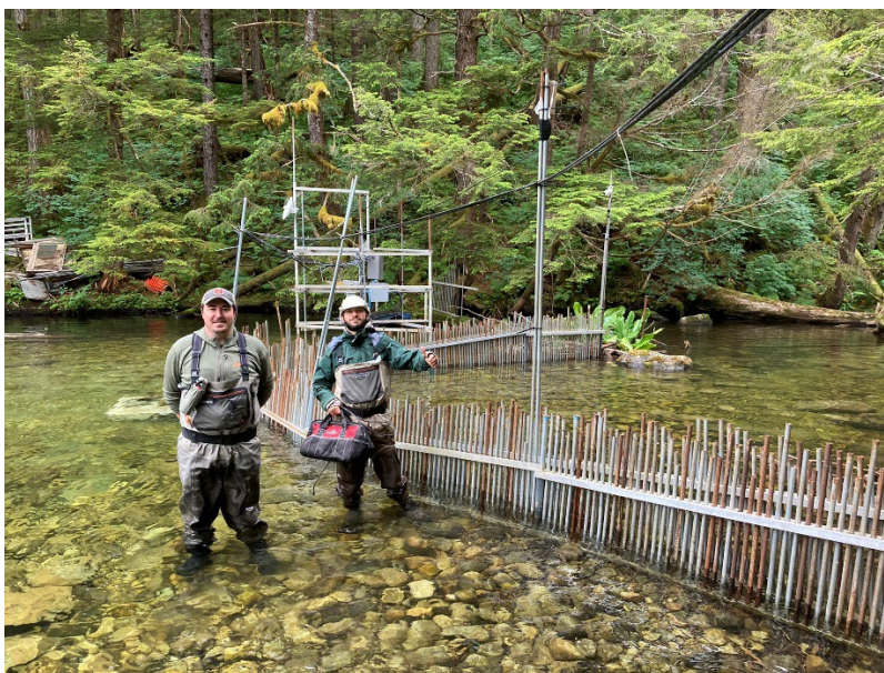
Figure 3. Taylor Cunningham (left) and Elijah Blumenkranz in front of the newly installed Neva Lake weir, June 18, 2022.
