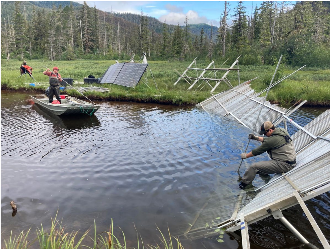
Figure 2. Matt Swifi (left, in boat) and Taylor Cunningham installing the Sitkoh Lake weir, July 14, 2022.
