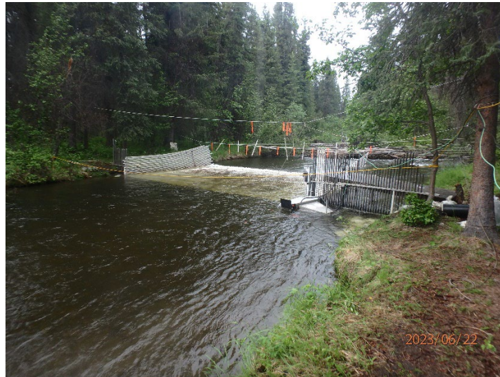
Tanada Creek Salmon Weir, 2023
