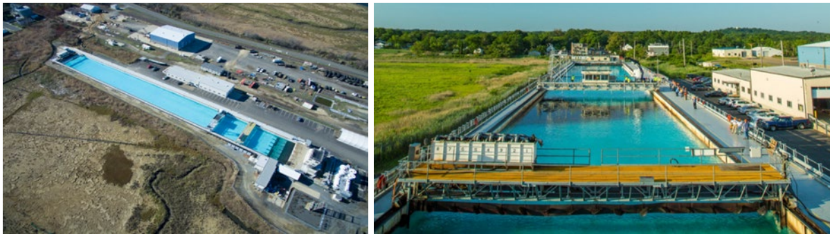
Figure 2: Overhead (left) and tank-level views (right) of the Ohmsett Facility in Leonardo, New Jersey.
