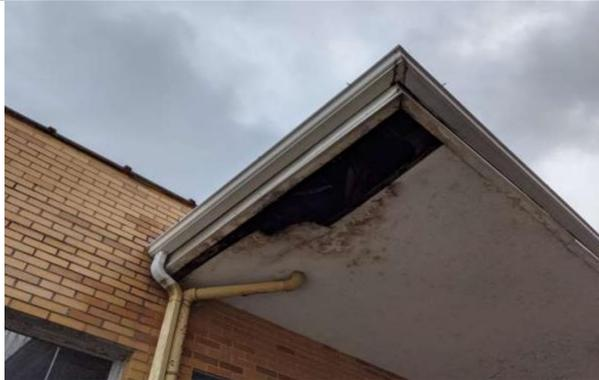
Greyhound Bus Depot, south canopy roof soffit showing deterioration.
