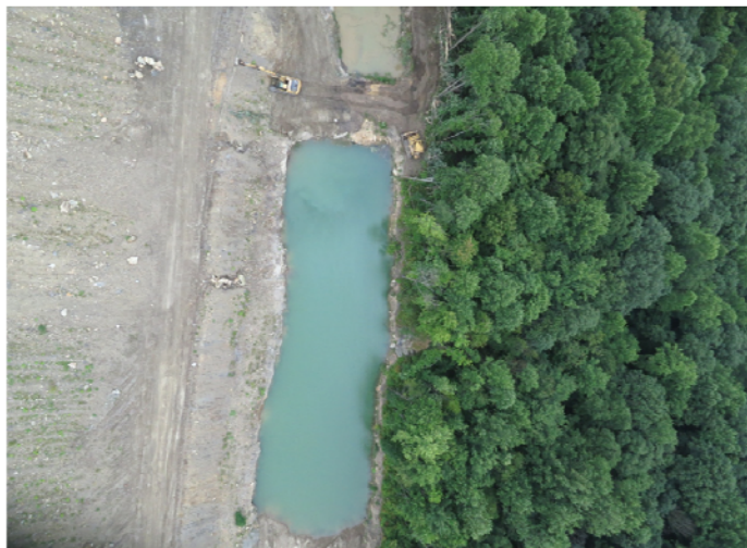
A perimeter pond at a surface coal mine in Bell County, Kentucky, as seen from above with RQ-16A T-Hawk. The outlet does not appear to discharge into a natural or designed channel as required. This information would prompt an onsite inspection. Photo was taken for OSMRE by the T-Hawk, remotely piloted by Lance Brady, BLM.
