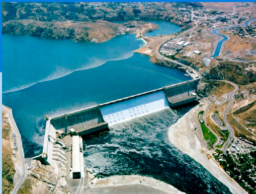
Grand Coulee Dam, USBR
