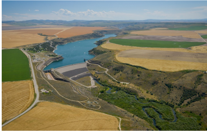
Ririe Dam, Ririe, Idaho. [Photo: Kirsten Strough]
