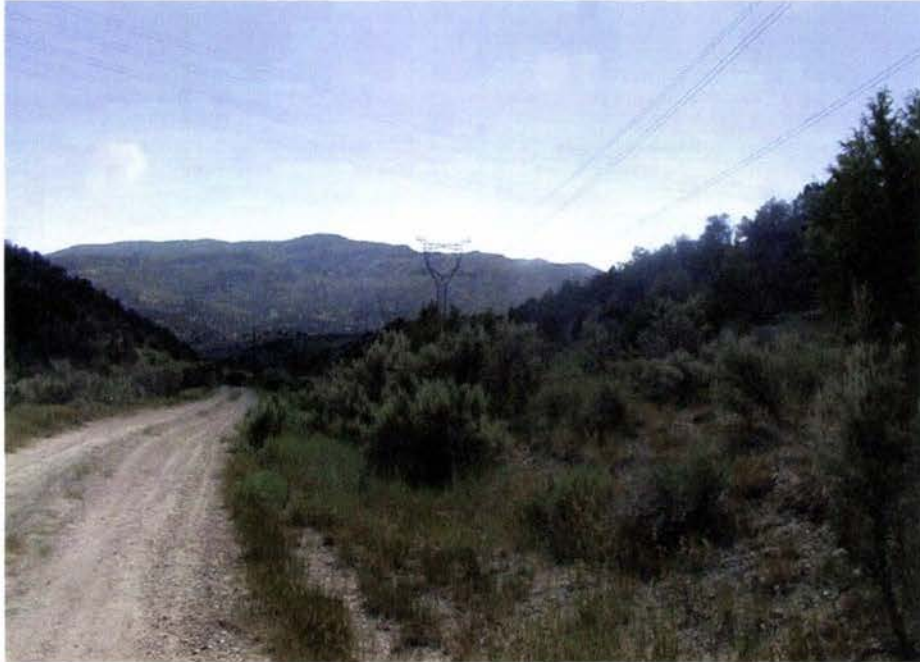
Photo No. 5 Looking South down Sheep Creek Road approximately 1 mile above Sub-station site
