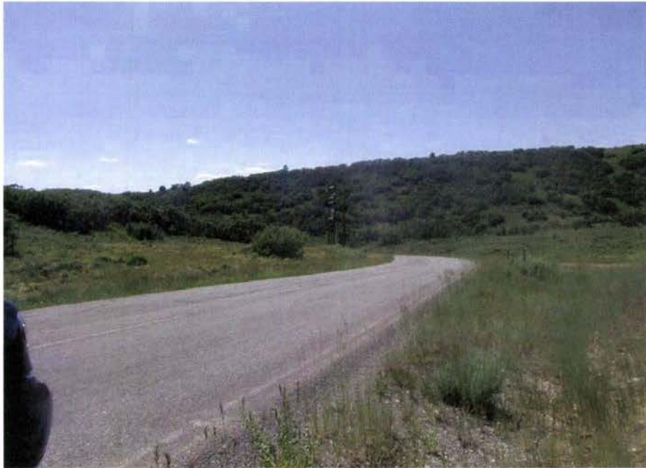
Photo No. 12 Power Line crossing Rays Valley Road at Milepost 6.5 looking west
