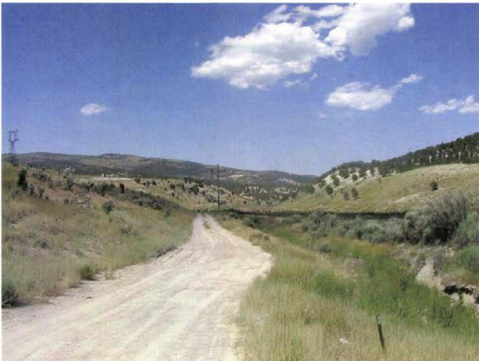
Photo No. 4 Looking North up Sheep Creek Road above Sub-station site
