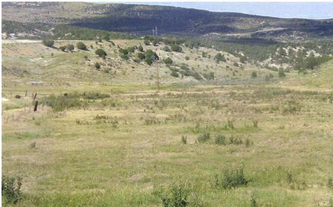
Photo No. 2 Sub-station site in Sheep Creek Valley above berm looking North
