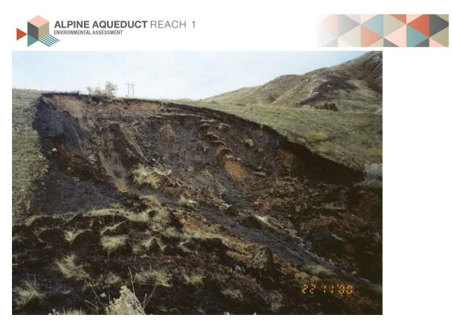
Figure 1-7. 2000 Landslide that Caused AA-1 Failure.
