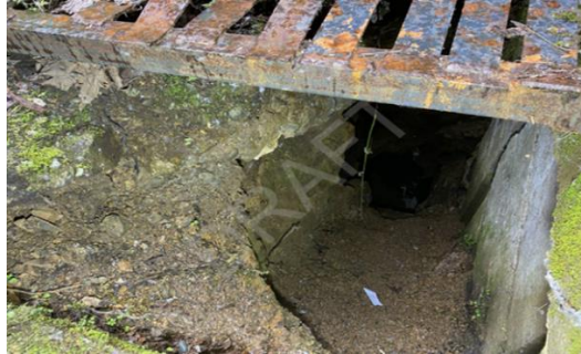
WA-21-002 Project: Vertical opening
