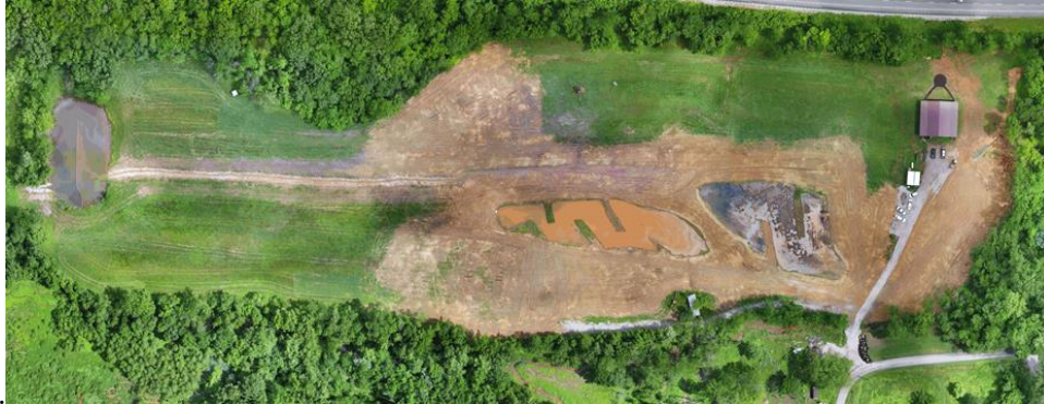
Sass Abatement Project, Ohio County, KY.
