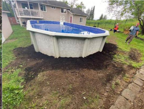
WA-21-005 Project: Site hazards mitigated, and pool reassembled
