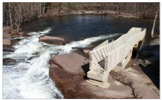
Partially completed Manhan River dam fishway in Easthampton, MA. Settlement funds from the Holyoke Gas Tar Deposits settlement contribute to the overall funds needed to complete the Denil fishway for anadromous fish passage. (Photo credit: FWS)
