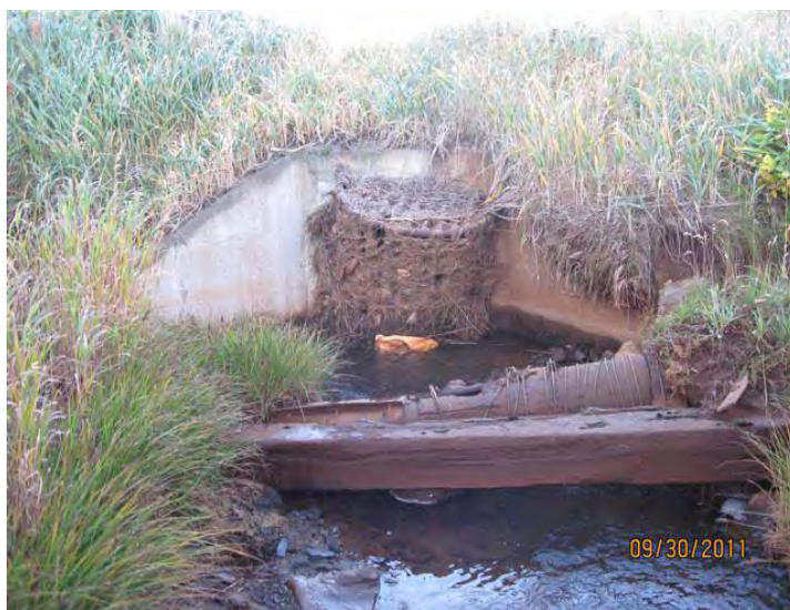
Figure 3: Wood stave pipe and timber
