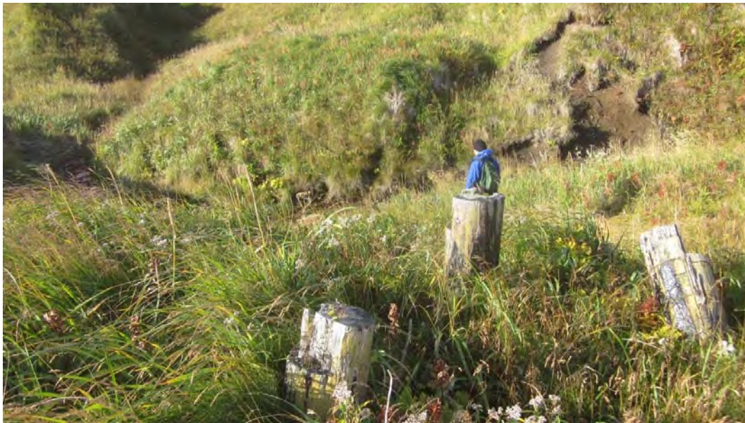
Figure 7: Upper Bank Pilings
