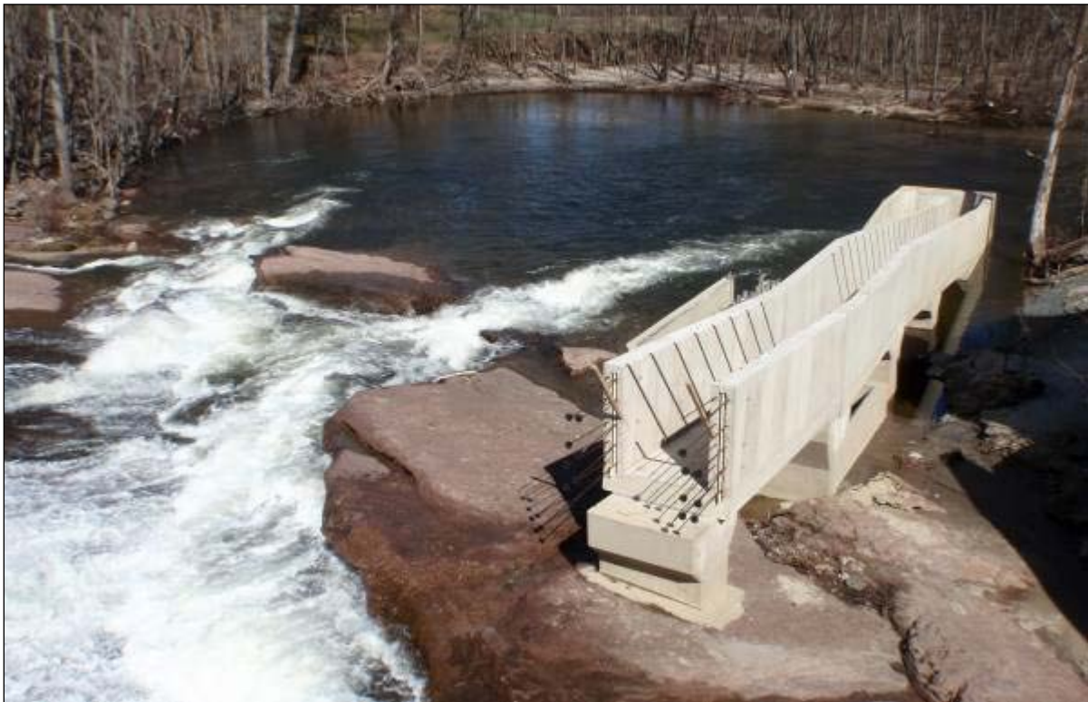
Figure 6. Partially completed Manhan River dam fishway in Easthampton, MA. Settlement funds would contribute to the overall funds needed to complete the Denil fishway for anadromous fish passage.
