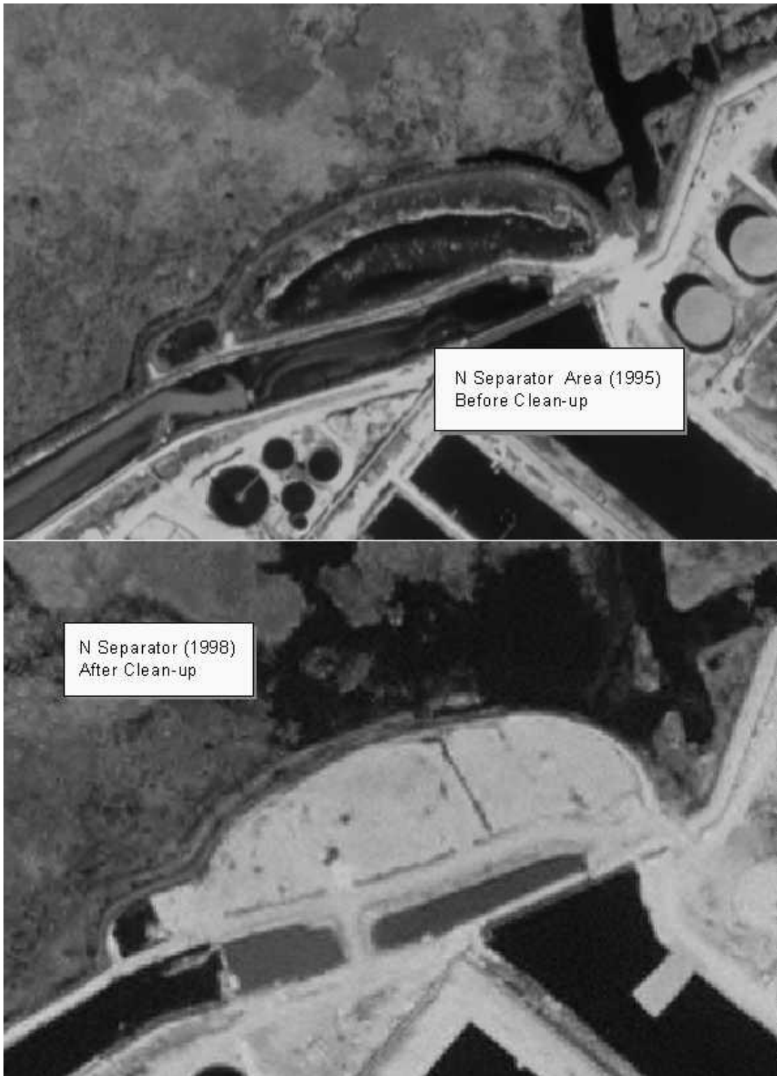
Figure 2.2 Example of complete corrective measures construction, North Separator Area, Old Gulf Oil Refinery Site, Jefferson County, Texas
