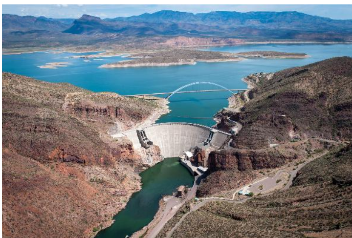
Theodore Roosevelt Dam and Bridge, Salt River, Arizona. This Dam, originally completed in 1911, was the first multipurpose project built by the Bureau of Reclamation. The bridge was added and the Dam renovated and expanded between 1986 and 1996. Photo: Bureau of Reclamation. Photographer: Andy Pernick.
