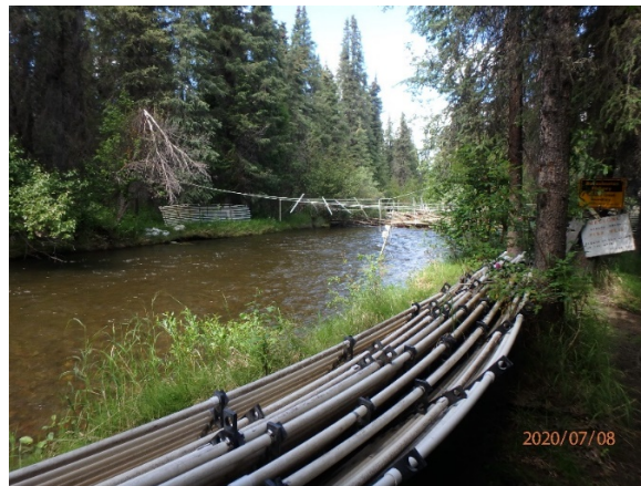
Photo of Tanada Creek weir site.
