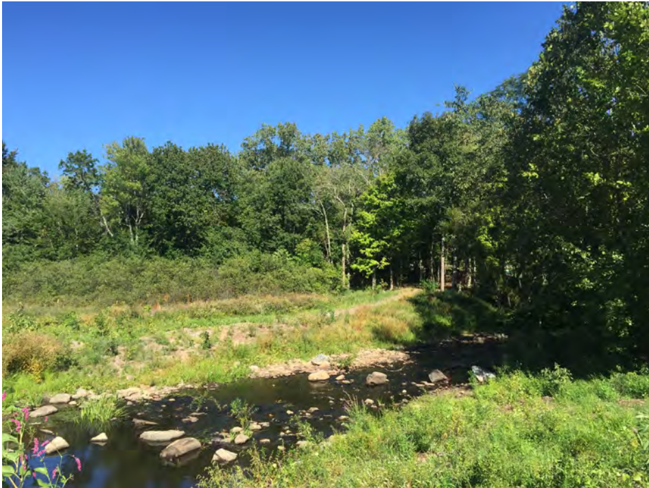
Pond Lily Dam removal, Connecticut. Photo credit: Save the Sound
