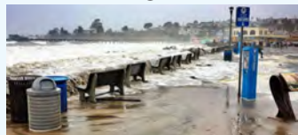
Along the southern end of Ocean Beach, San Francisco, California, the bluff severely eroded the shoreline 55 meters during the winter 2009–10 El Niño season, including this damage along coastal California's Highway 1. Photo credit: Jeffrey Hansen, USGS
