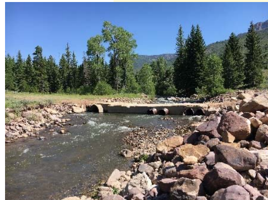
Existing River Crossing Structure
