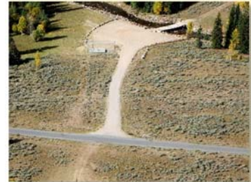
Existing North Fork Siphon Blow Off Structure with existing river crossing in the background
