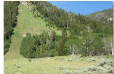
Overview of the area of the construction access road to the Hades Inlet Tunnel Portal looking west
