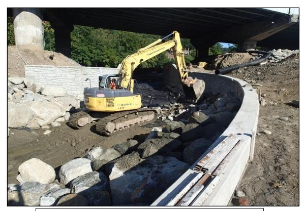
Construction of bypass channel at the Tingue Dam. (Photo by CT DE&EP)
