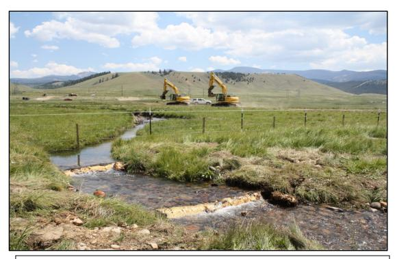
Construction activities at the upper Arkansas River excavated pools, created stream riffles, and added woody debris and boulders to create improved feeding and spawning areas in the river. (FWS photo)
