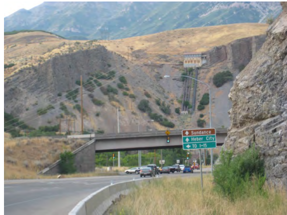
View of Pressure Box just prior to entering Provo Canyon
