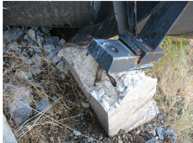
Displaced support
