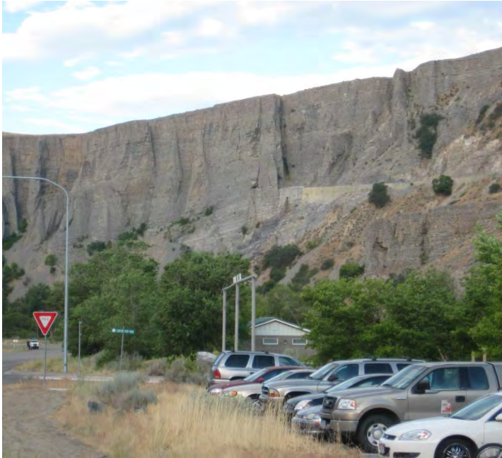
View of the Encased Pipeline with Spillway from US-189
