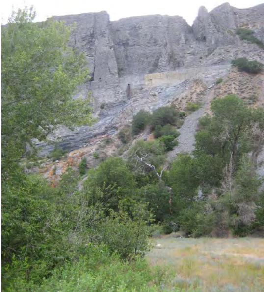
View of the Pipeline Encasement and Spillway from the Provo River Parkway Trail
