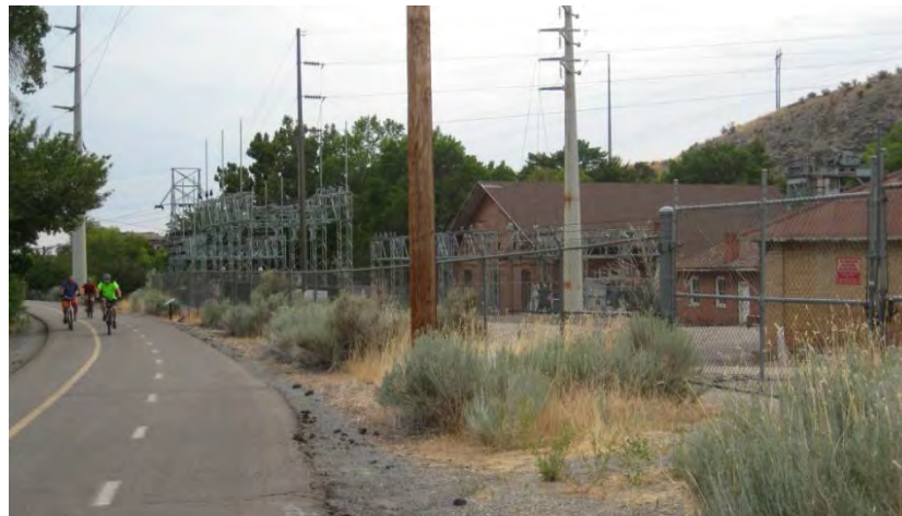
View of Olmsted Power House and Auxiliary Buildings from the Provo River Parkway Trail
