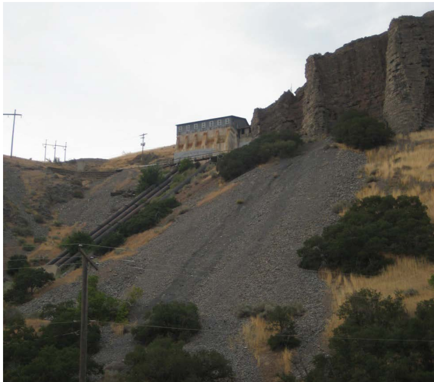
View of the pressure box from the Provo River Parkway Trail
