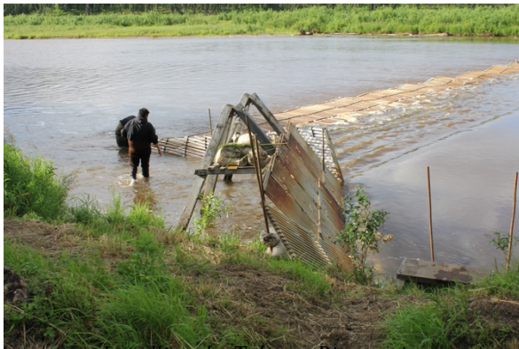
Installing the Takotna River weir.
