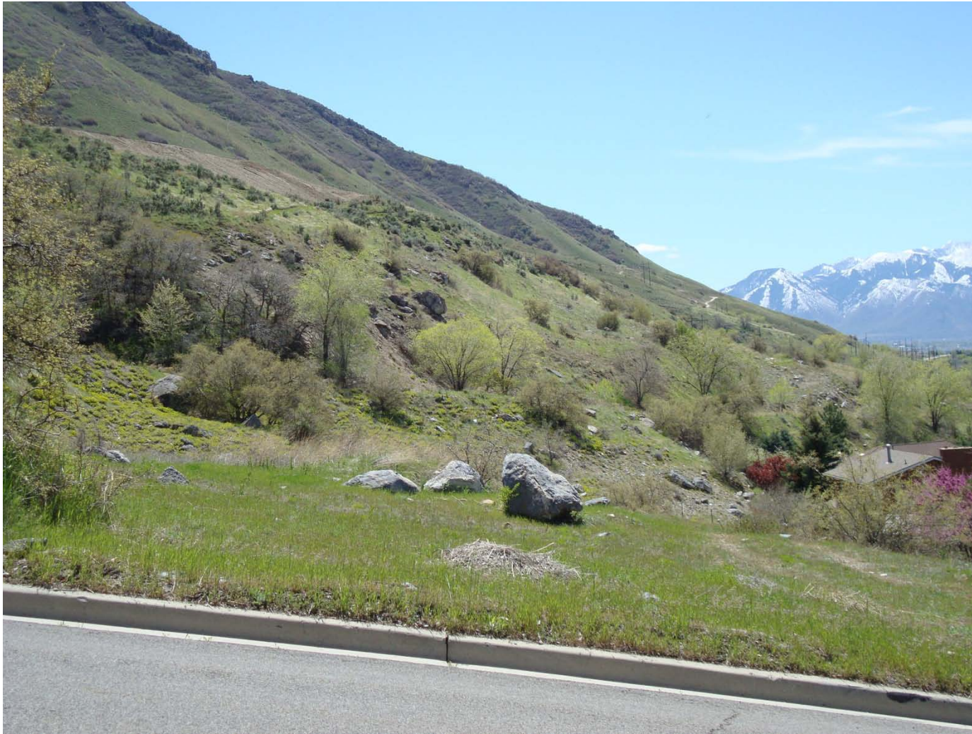
Photo 1: Looking at toe of existing steep slope between approximate DPR stations 688+00 and 705+00, from a point west and down slope of approximate station 705+00. The DPR alignment crosses the lower portion of this slope, above the house at the far right of the photo.
