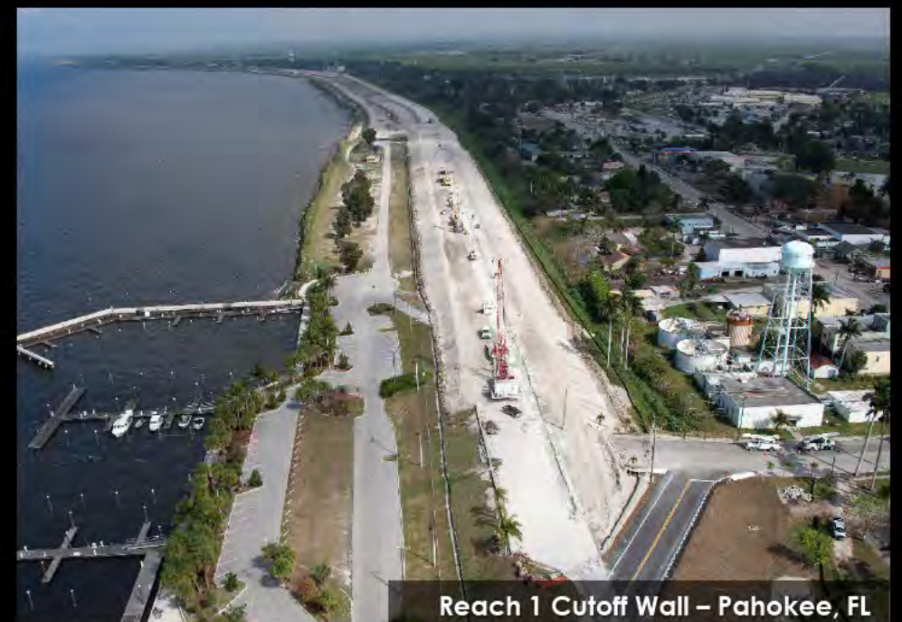
Reach 1 Cutoff Wall – Pahokee, FL
