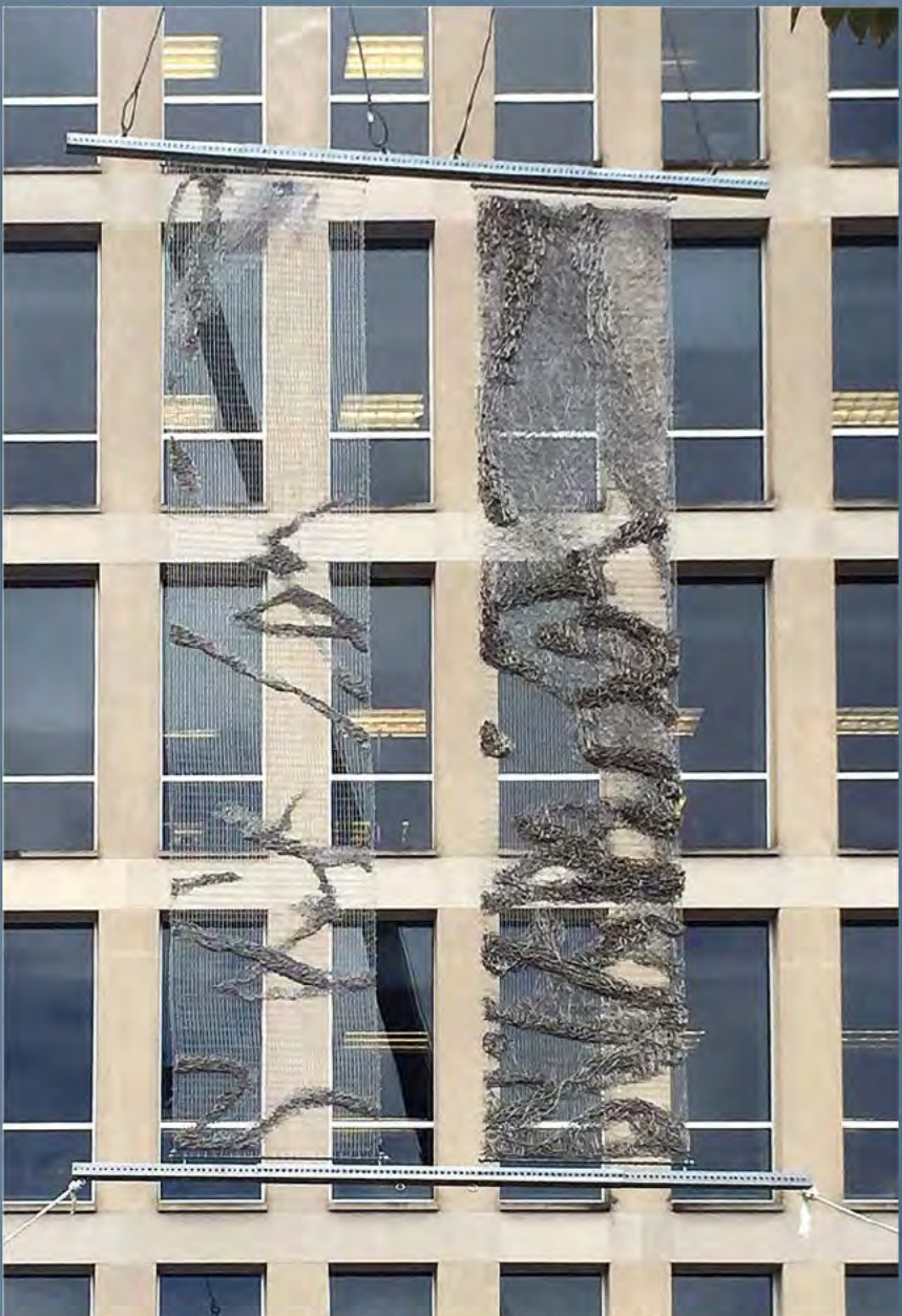
Looking south to the LBJ Building
