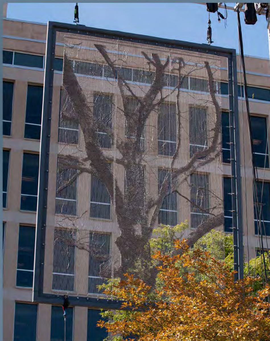
Looking south to the LBJ Building
