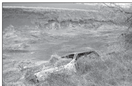
Source: GAO. Abandoned Car in Canal
