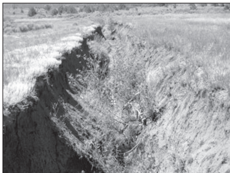
Irrigation Ditch in Need of Reshaping
