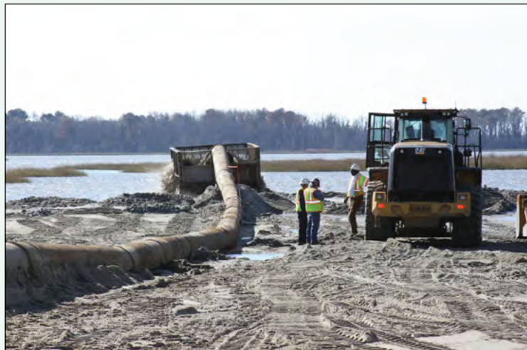
Pumping sand operations to restore beach, dunes and close breaches at the Prime Hook Refuge. Photo credit: Tim Boyle, USACE
