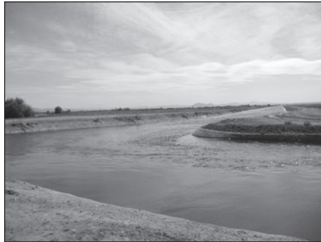
Source: GAO. Concrete-lined Irrigation Canal
