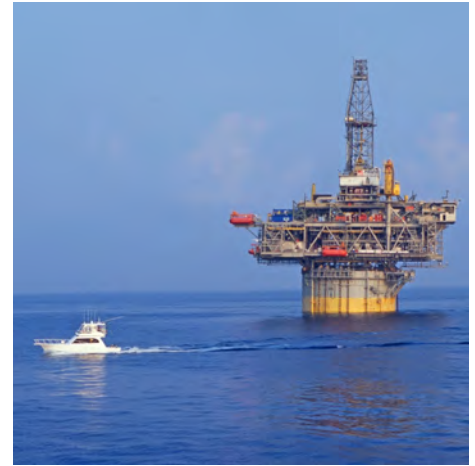
The Mad Dog platform is a floating spar facility in the Gulf of Mexico. Photo credit: BP
