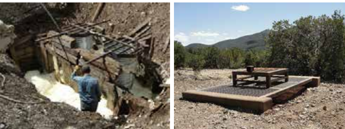
San Pedro - Polyurethane foam closure under construction San Pedro - Completed bat cupola
